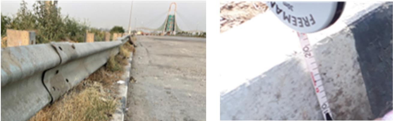
**Figure 5. High median and raised kerb in front of crash barrier (responsible for single vehicle overturning and tyre burst)**
